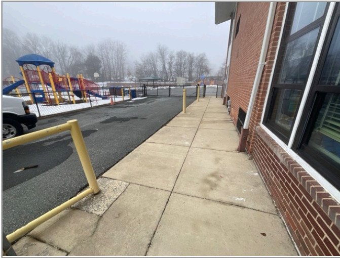
ACCESSIBLE ROUTE TO PLAYGROUND
