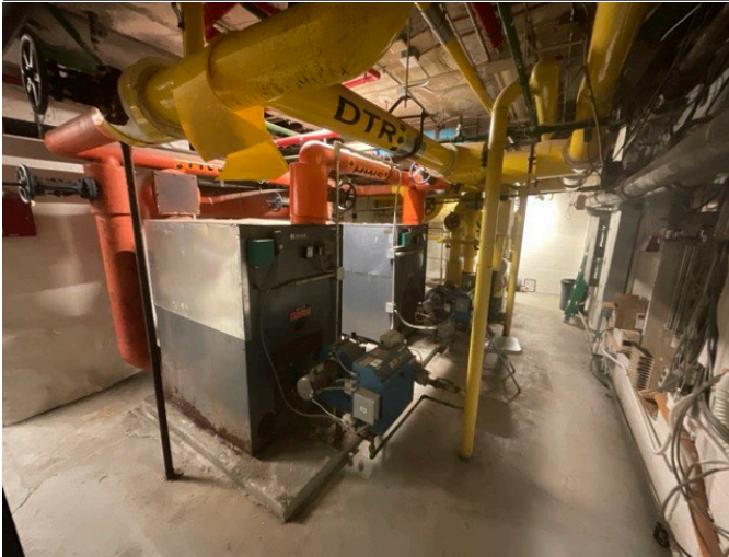
7 - OLD BOILER ROOM
