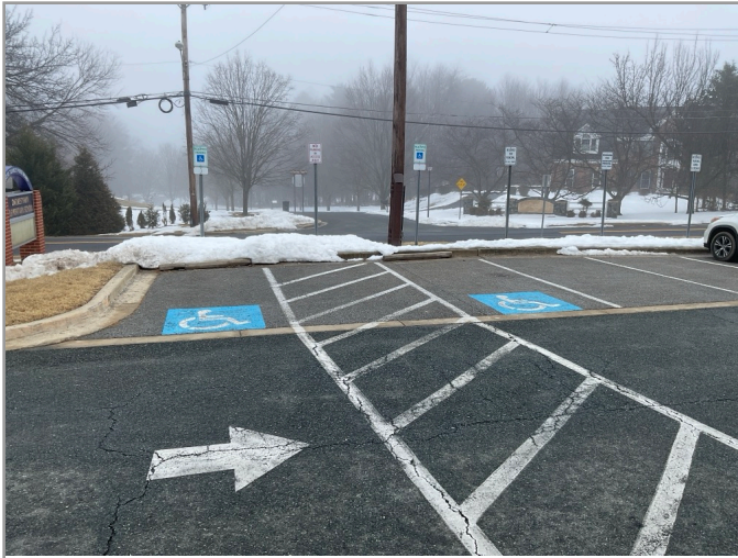
OVERVIEW OF ACCESSIBLE PARKING AREA
